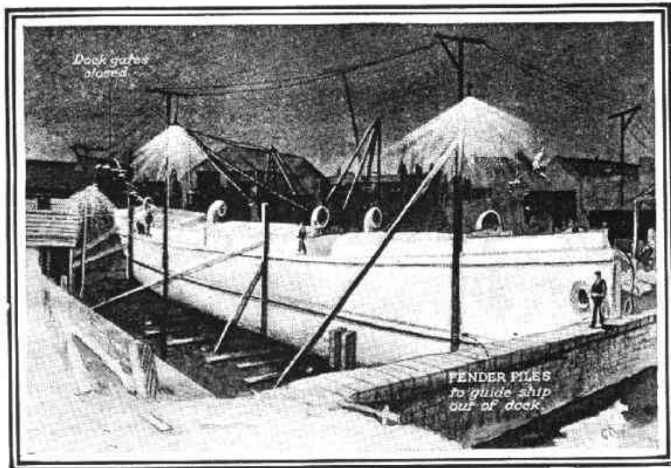
(5) The Finished 900-ton Vessel in Dry Dock
